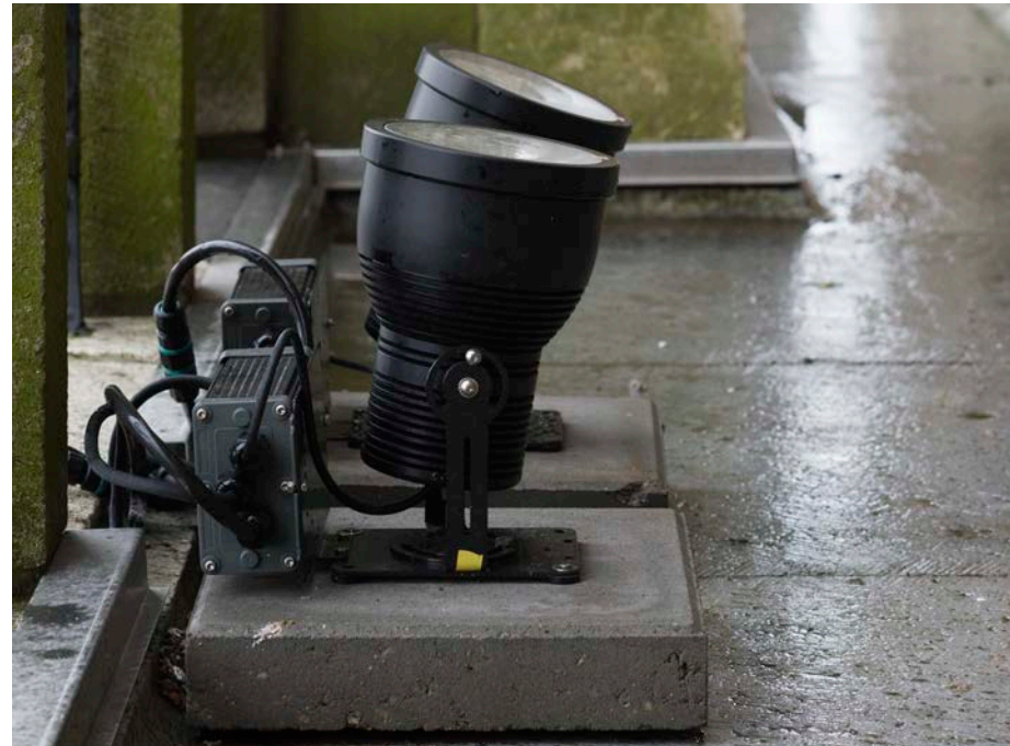
Dom Tower, Utrecht, lighting fixed onto concrete slab to avoid damage to the fabric.
