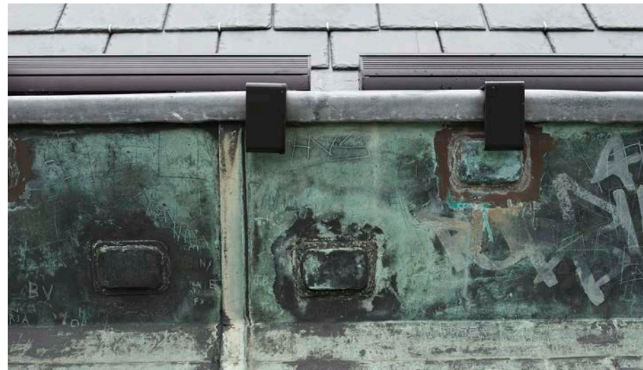
Dom Tower, Utrecht, lighting fixed onto concrete slab to avoid damage to the fabric.
